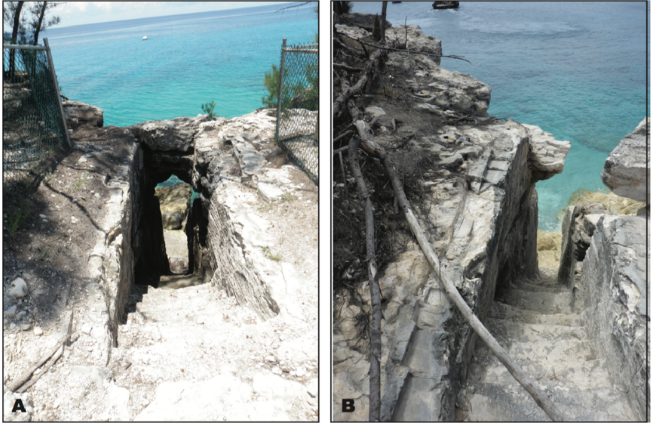
Figure 8: The Pirate Stairs near Clifton Pier showing damage from Hurricane Matthew. A) Photograph from June 2012, and B) Photograph from March 2017. Note the fence that once stood at the edge of the cliff and around the stairs in the 2012 image and the broken and transported lintel block.
