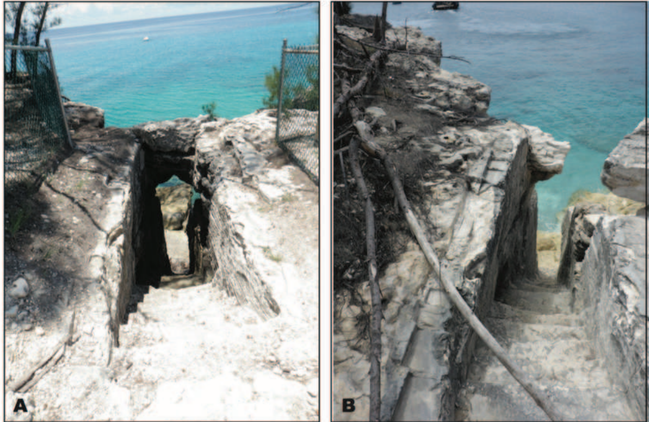
Figure 8: The Pirate Stairs near Clifton Pier showing damage from Hurricane Matthew. A) Photograph from June 2012, and B) Photograph from March 2017. Note the fence that once stood at the edge of the cliff and around the stairs in the 2012 image and the broken and transported lintel block.
