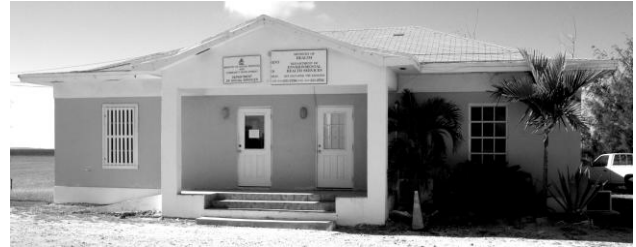
Figure 26. The building housing the San Salvador offices of the Bahamas Department of Environmental Health and Department of Social Services is depicted in this image from 2011.
