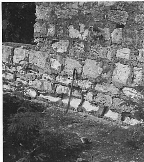
Figure 5. Tafoni (arrows) in eolian calcarenite quarried rock for building blocks for colonial period buildings, Watlings Castle, San Salvador Island, Bahamas.
