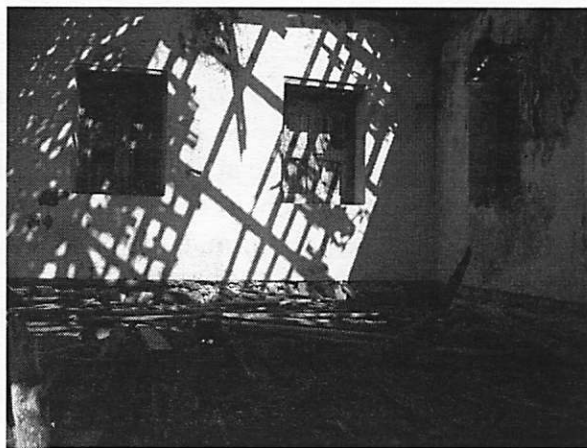
Figure 6: Queen's Highway Building 4, Polly Hill Settlement
