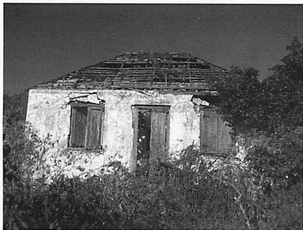
Figure 4: Queen's Highway Building 1, Polly Hill Settlement
